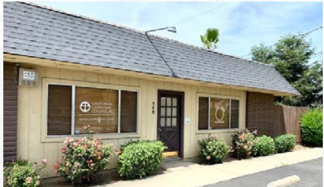
OFFICE BUILDING LOCATED ON WEST CALDWELL AVENUE
